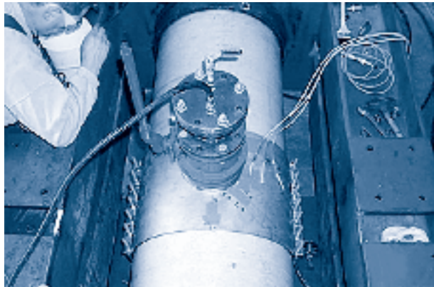
Figure 8-2 Pressure testing of sleeve and valve assembly
