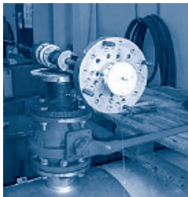
Figure 8-3 Tapping machine, valve and retrieved coupon
