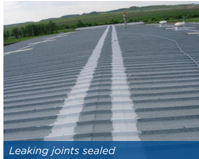
Full roof encapsulation
