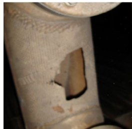
Damage to pipework
