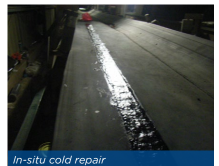
Internal section lined with Belzona
