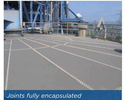
Base sealed with a Belzona coating
