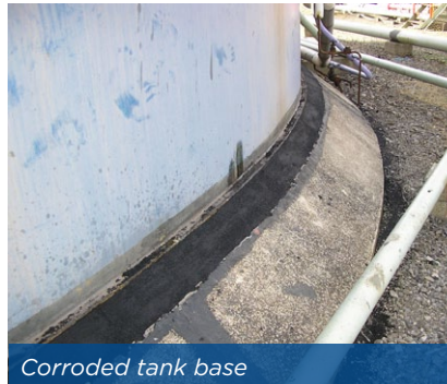
Corroded tank base
