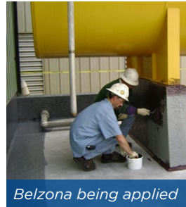
Concrete rebuilt
