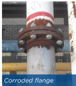
Severely corroded pipe
