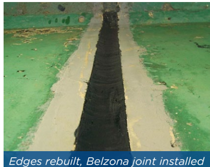
Edges rebuilt, Belzona joint installed
