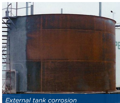
Corrosion at joints on storage tank
