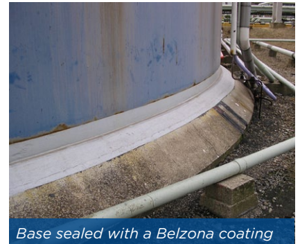
Base sealed with a Belzona coating
