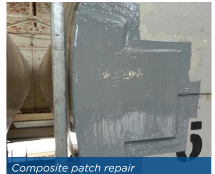
Joints fully encapsulated
