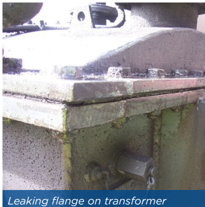
Transformer leaking oil from cracks
