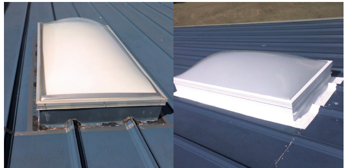
Skylights sealed with waterproofing membrane
