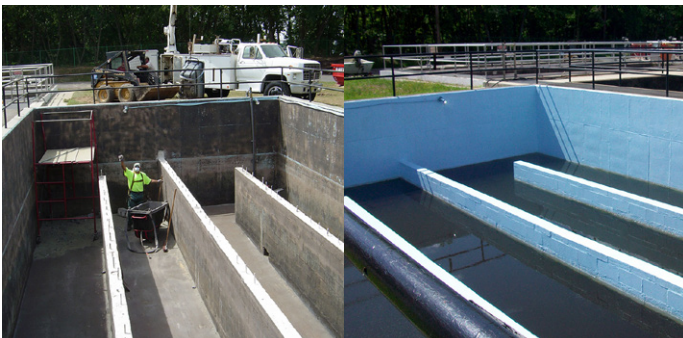
Chlorine tank protected against chemical attack
