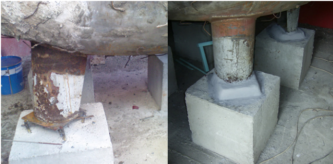
Vessel supports reconstructed
