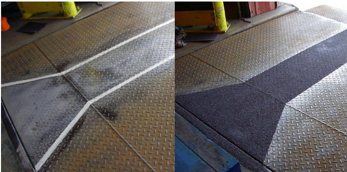
Safety grip system applied on loading bay
