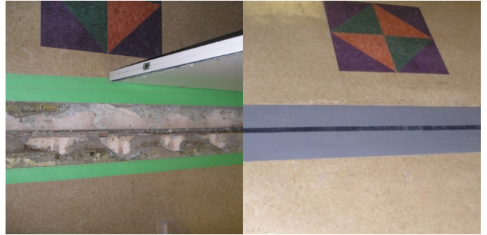
Failed expansion joint in hospital repaired
