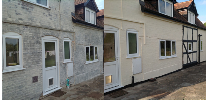
Deteriorated wall protected from water ingress
