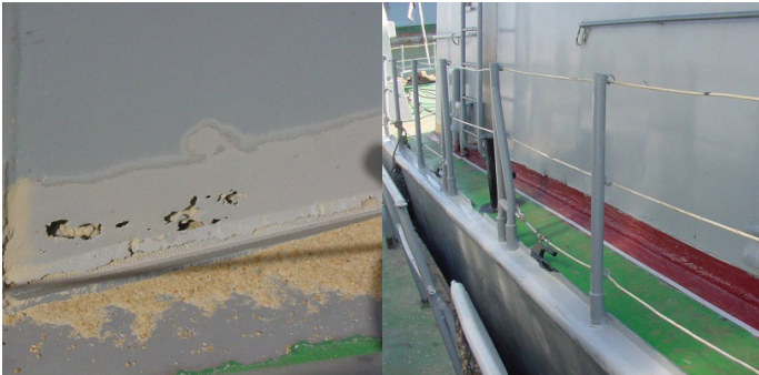
Joint between deck and vessel sealed
