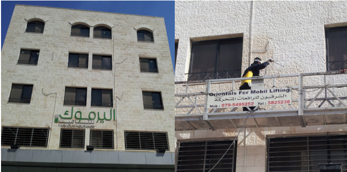
Clear water repellent treatment applied to masonry wall
