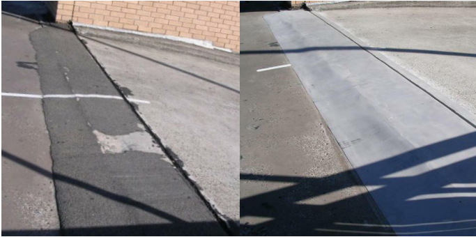
Expansion joint sealed
