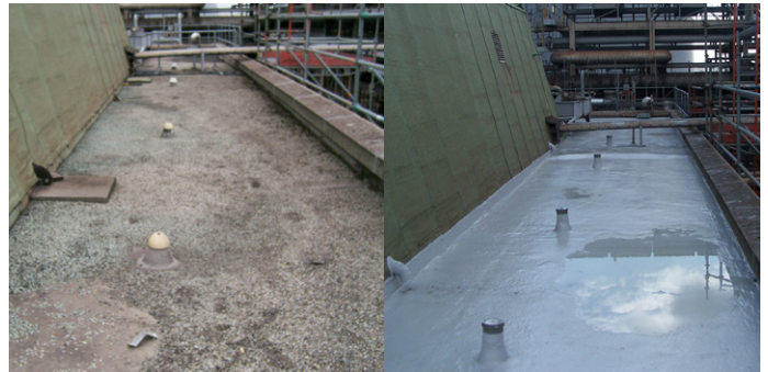
Sealed flashing at roof/wall interface
