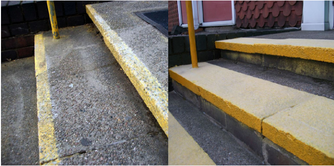
Safety grip system applied on concrete steps
