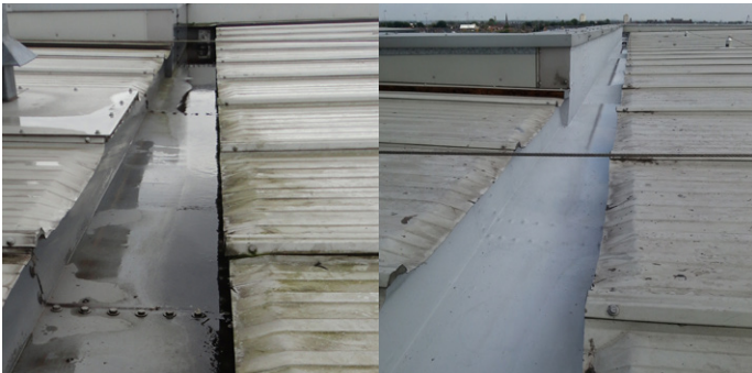
Damaged gutter seamlessly sealed
