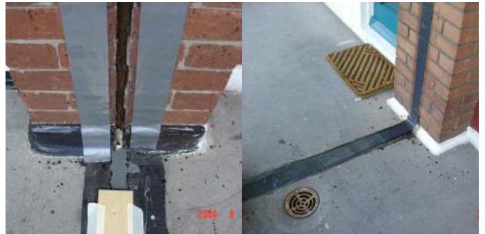
Leaking expansion joint repaired
