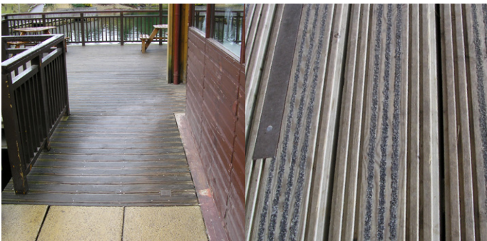
Safety grip system applied on decking
