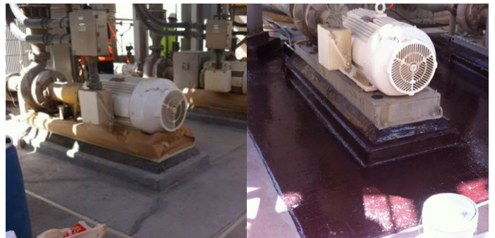
Containment area protected against chemical attack
