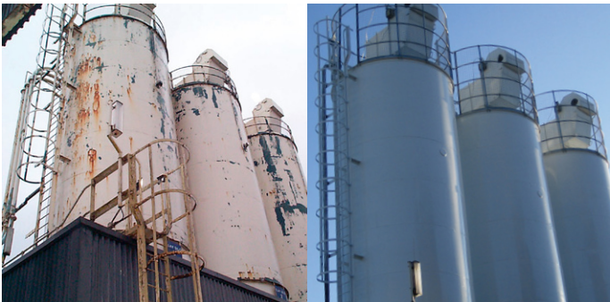
Robust long-term coating of sugar silos
