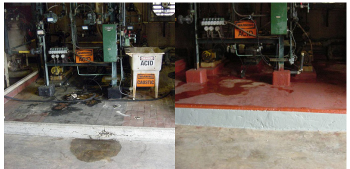
Chemical handling area resurfaced
