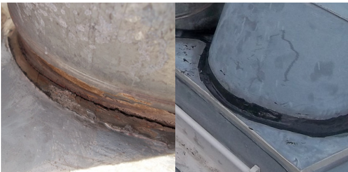
Deteriorated HVAC joints sealed
