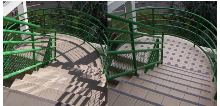
Safety grip system applied on tile staircase
