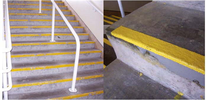
Worn step nosings rebuilt
