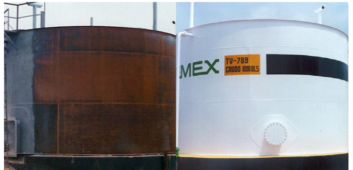
Storage tank protected from external corrosion
