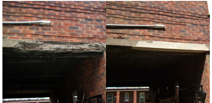
Overhead lintels repaired
