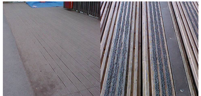
Safety grip system applied on wooden bridge
