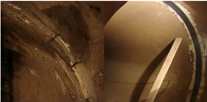
Joints sealed on underground concrete pipes
