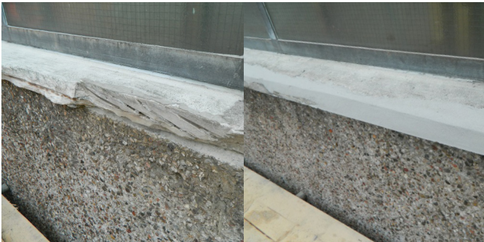
Spalled concrete window sill repaired
