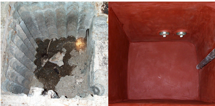
Sump rebuilt with chemically resistant material
