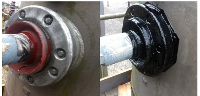
Fully encapsulated flange
