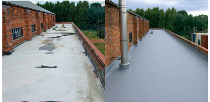
Deteriorated asphalt roof waterproofed
