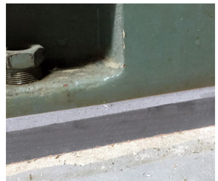
Precise alignment of the equipment
