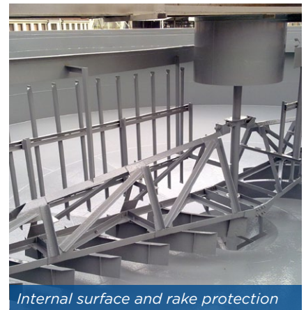
Completed lining application
