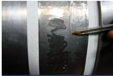
Worn out shaft
