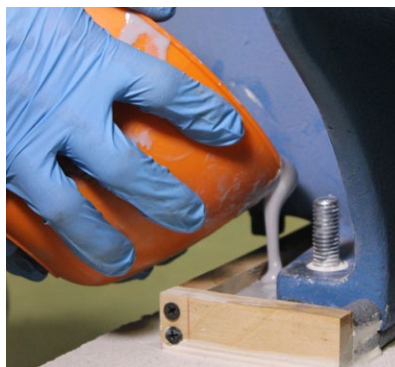
Chocking in progress
