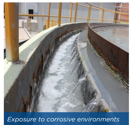
Equipment under chemical attack
