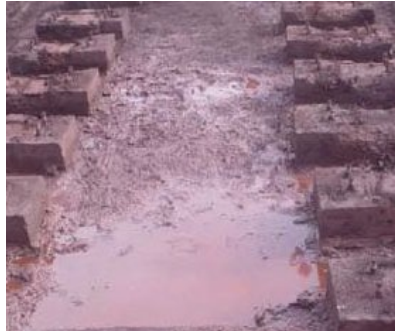
Damaged bases of railroad tracks
