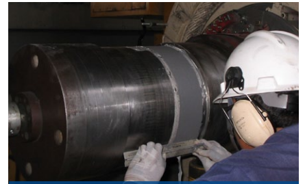
Shaft rebuilding in progress
