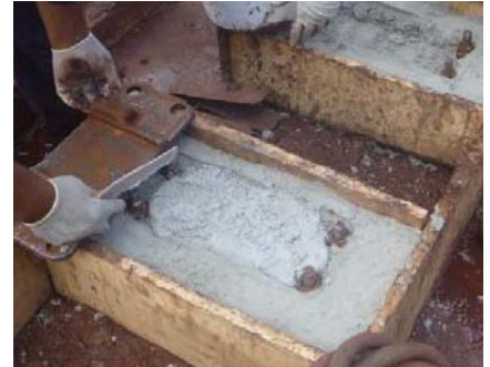
Restoration in progress
