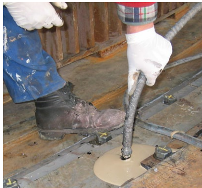
Shimming excavator bearing seats
